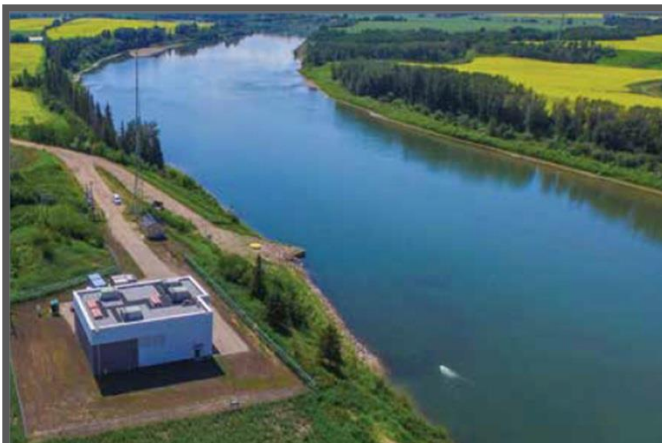
INDUSTRIAL WATER SERVICES CANADA 85,200 m 3 /day
