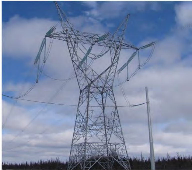
FORT MCMURRAY WEST 500 KV TRANSMISSION
