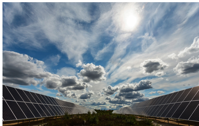
Old Crow Solar Project - Old Crow, Yukon
