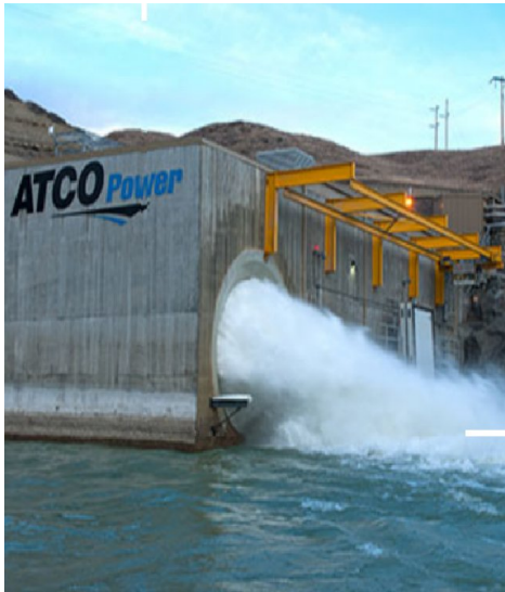
Oldman River Hydroelectric Plant
