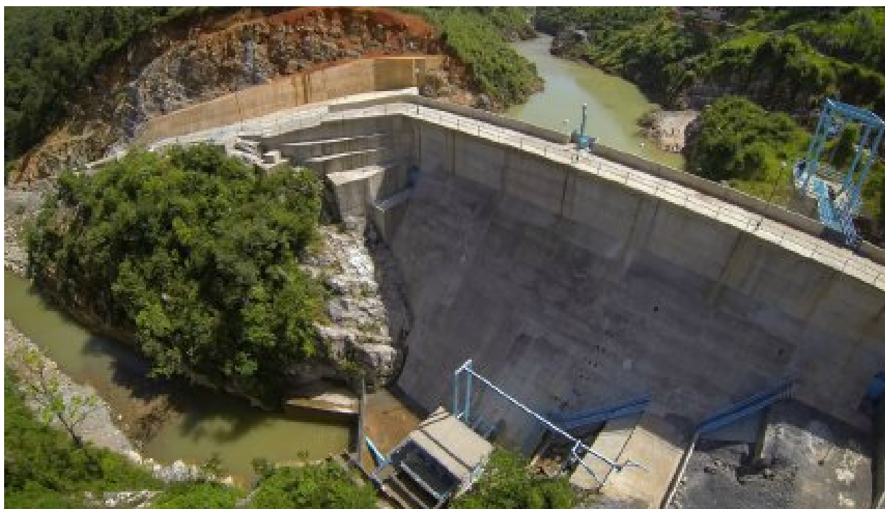
Electricidad del Golfo Hydroelectric Power Station
