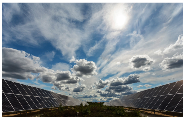
Old Crow Solar Project - Old Crow, Yukon
