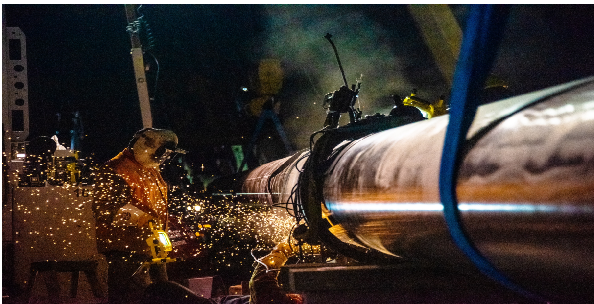
Pembina-Keephills transmission pipeline construction, near Wabamun Lake, Alberta
